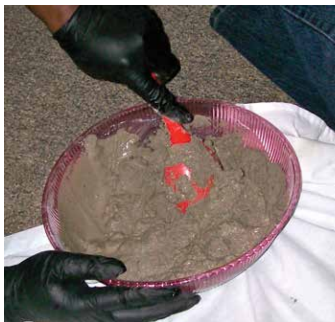
Mixing mortar by hand
